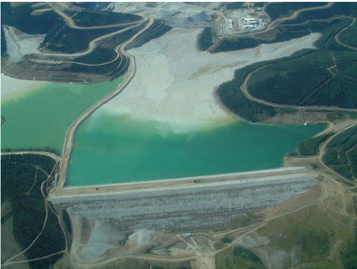
TAILINGS DAM AT FORT KNOX GOLD MINE — Mine tailings dam at Fort Knox ( /Issues/MetalsMining/FortKnoxMine.html ) gold mine with the mill facility in the background. — Get Photo ( /photos/tailings-dam-at-fort-knox-gold-mine/ )
