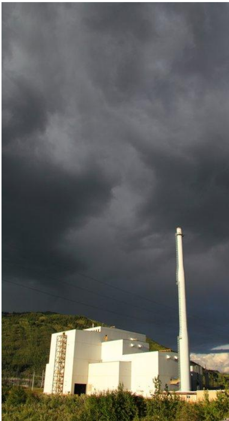
HEALY CLEAN COAL PLANT — This long idle coal power plant was state of the art when it failed to begin full-time operation in 2000. — Get Photo ( /photos/healy-clean-coal-plant/ )
