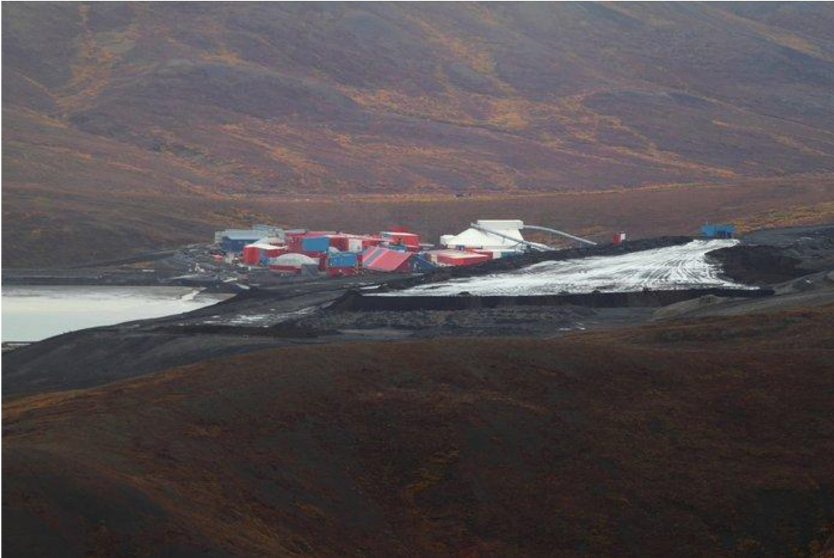
RED DOG MINE — Facilities situated between the tailings pond (at left) and the mine (not visible.) Waste rock piles are in the foreground. — Get Photo ( /photos/red-dog-mine_2/ )
