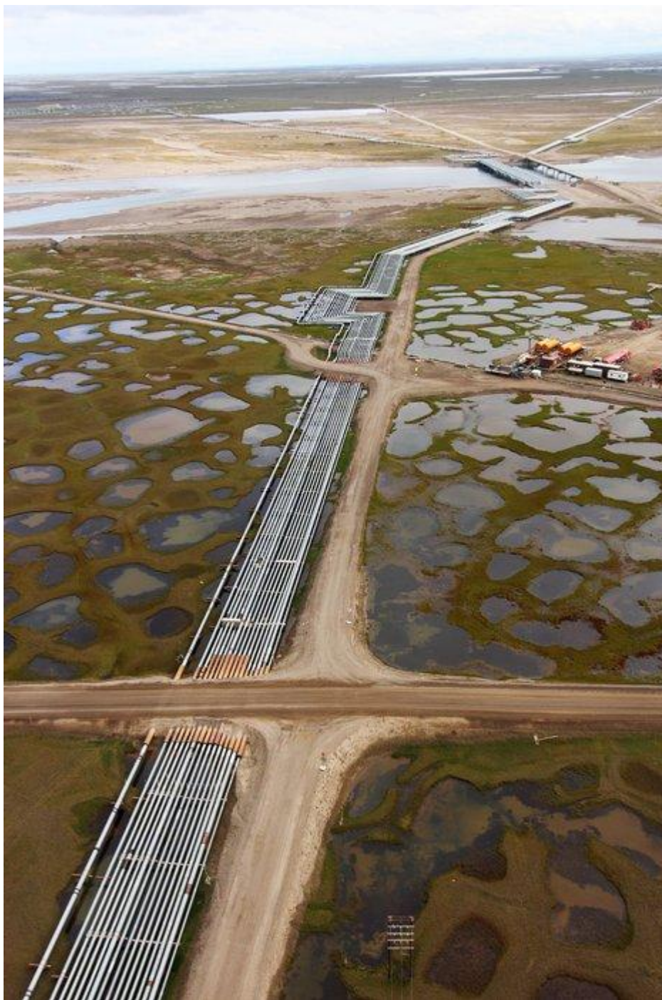
NORTH SLOPE PIPELINES — Pipelines crossing tundra west of Prudhoe Bay in Alaska’s Arctic. — Get Photo (/photos/north-slope-pipelines/)
